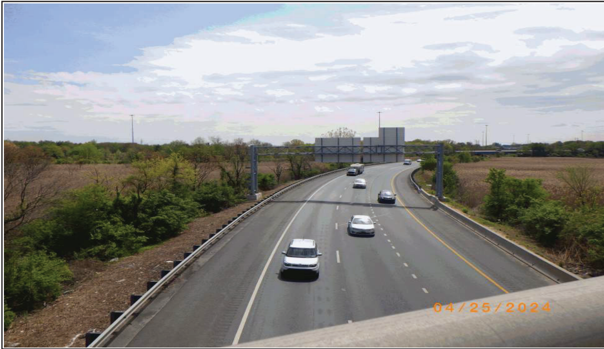
5 UNDER RECORD (SPAN 2 OVER I-95SB), LOOKING EAST
