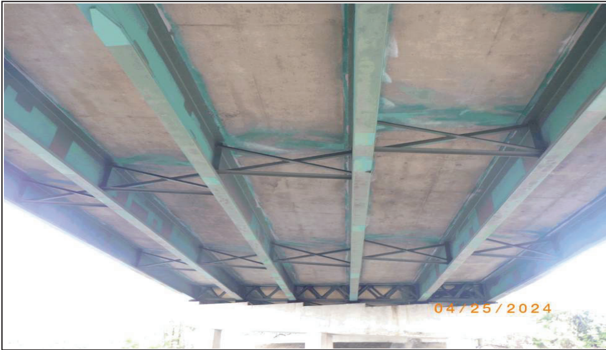
3 GENERAL VIEW OF SUPERSTRUCTURE (SPAN 2 SHOWN), LOOKING NORTH
