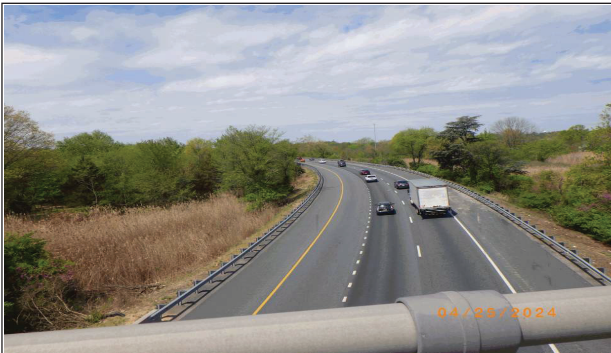
4 UNDER RECORD (SPAN 2 OVER I-95SB), LOOKING WEST
