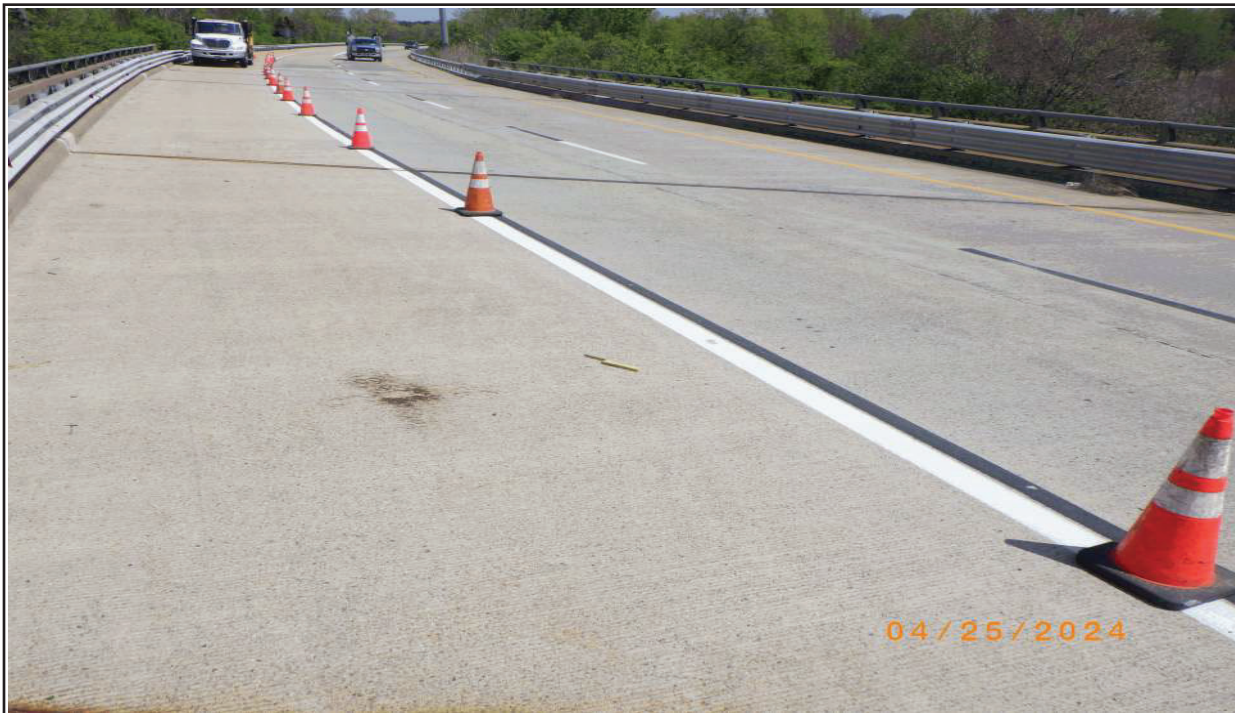
6 GENERAL TOP OF DECK (SPAN 1 SHOWN), LOOKING NORTH
