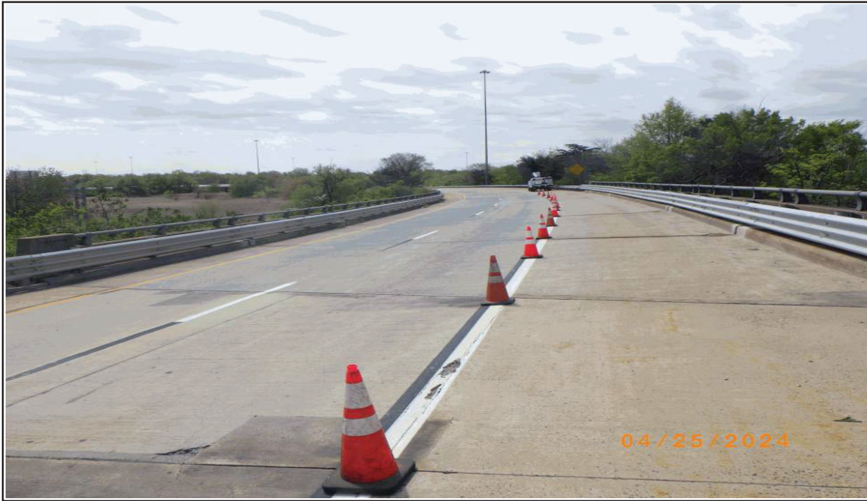
1 NORTH APPROACH, LOOKING SOUTH
